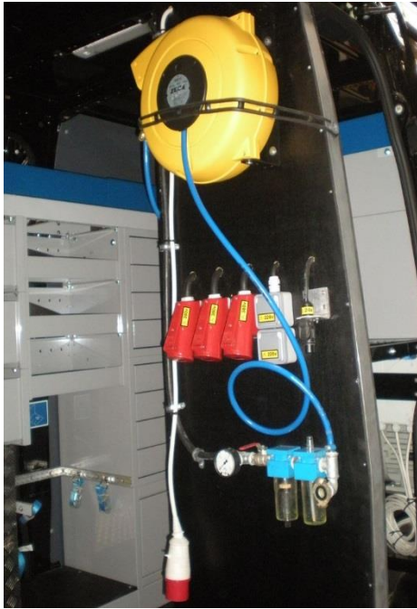
Welding equipment sockets
